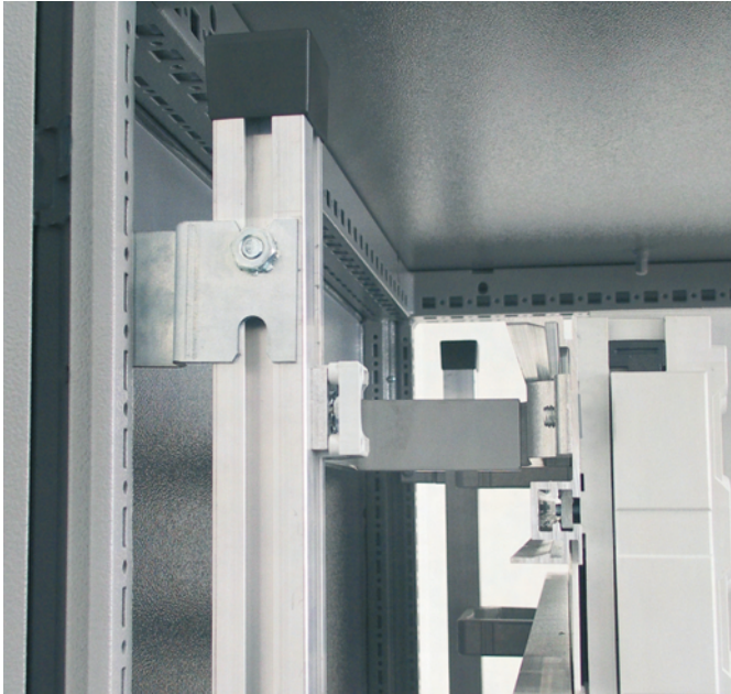
Installation of the LSC frame in the rearmost position with adapting brackets.
